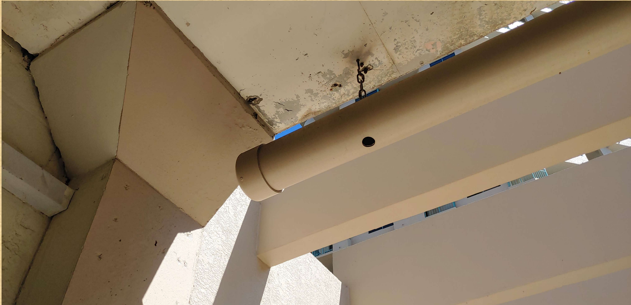
Exhibit H – Loading Dock Left Corner Missing Stucco
