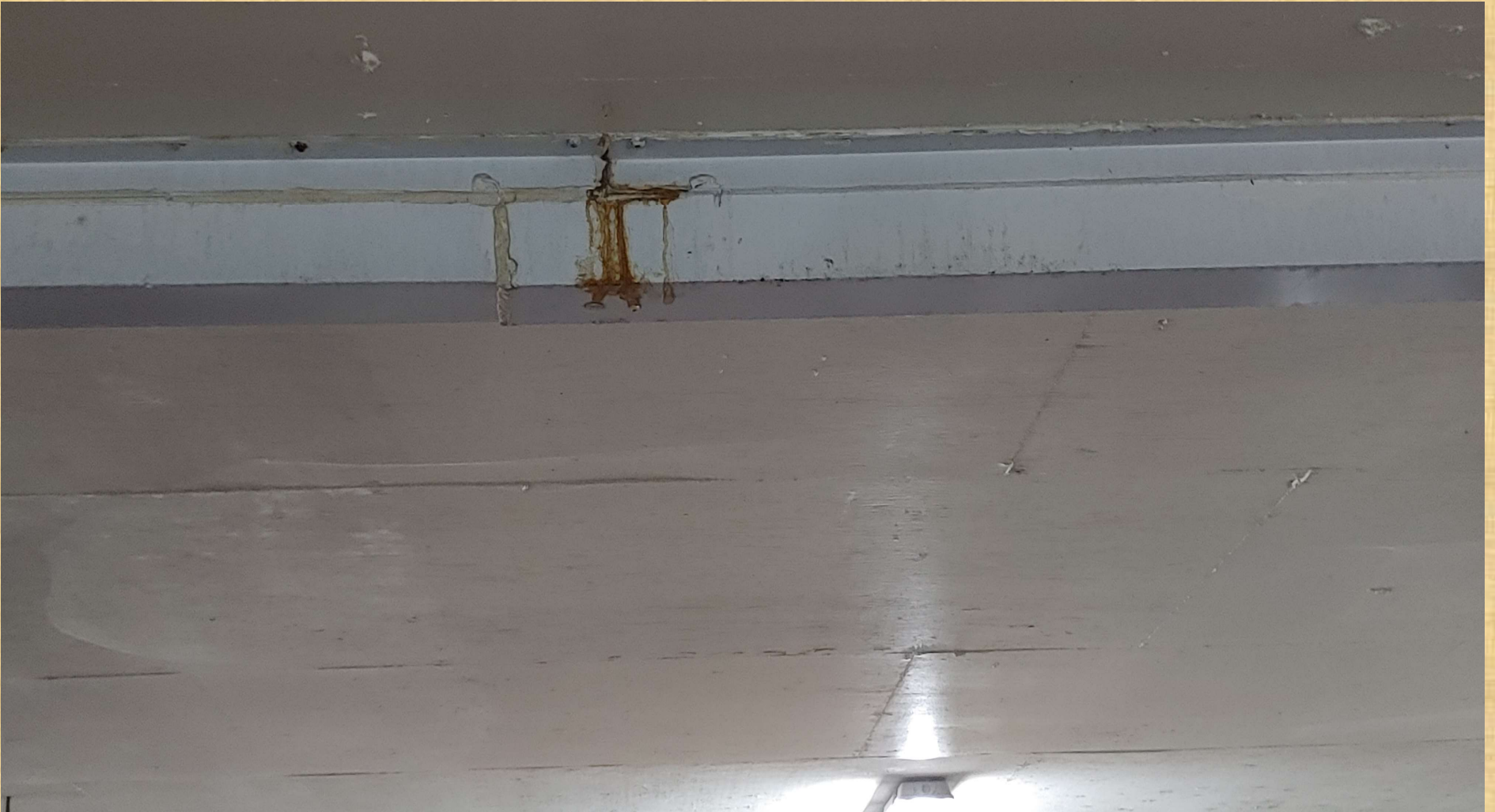
Exhibit E – Water Leak Over Car by Bike Rack
